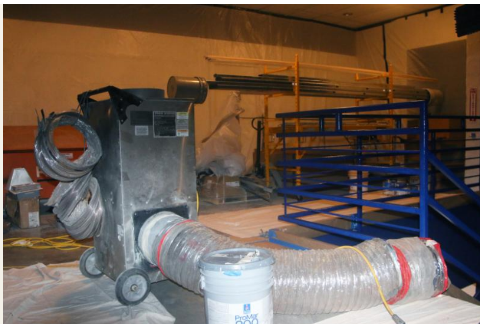
The HEPA vacuum used to catch construction dust in the gallery.
